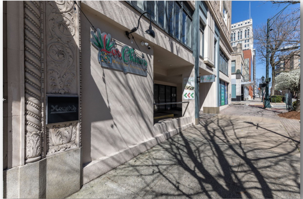
Building Entrance on Elm Street
